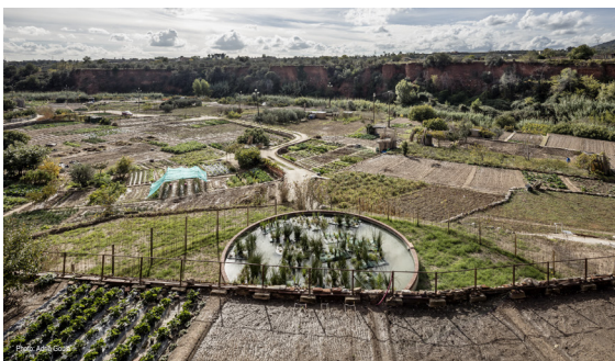
Pool current stage : public open space with the new pool integrated to the existing irrigation system to accumulate and cool the thermal water
